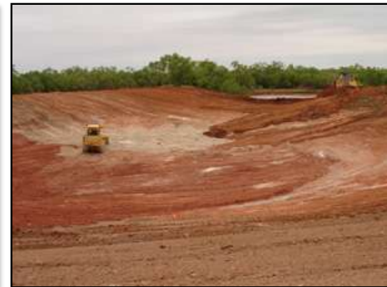
Initial lake construction
